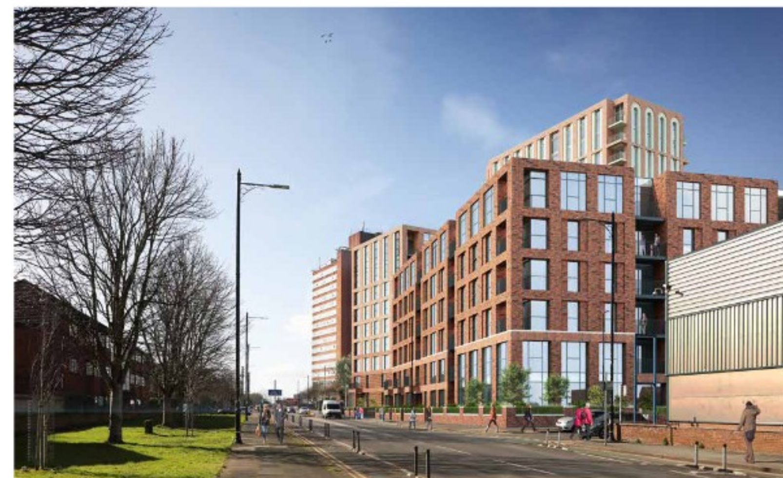
Stretford Road visualisation: Recessed balconies animate key corners and subdivide the facade
